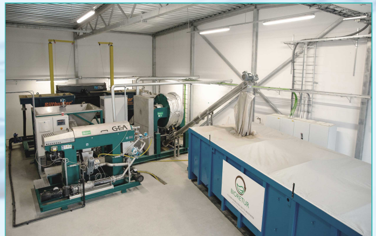
Photo showing installation of the award-winning FRS® Fish Sludge Recovery System operating at Erko Settefisk
